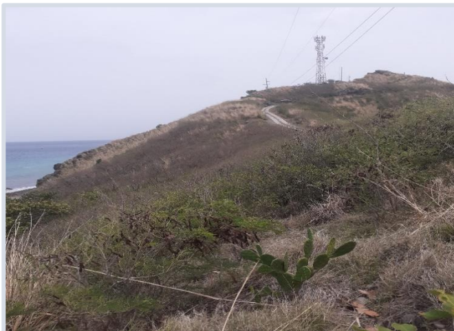
Figure 18 South Range damage-Scott's Head Peninsula, Sept. 2021
