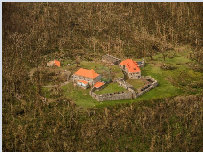
Figure 10 North Range-Cabrits National Park, Nov. 2017
