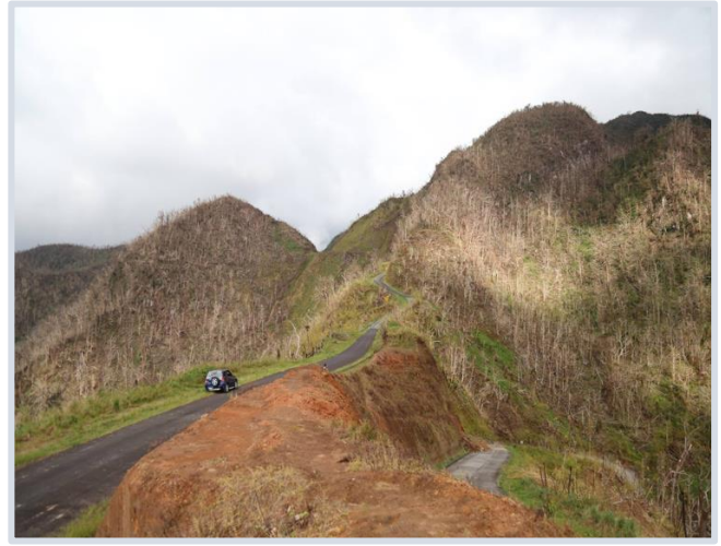
Figure 7 Northern Range damage, Nov. 2017
