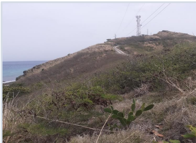
Figure 18 South Range damage-Scott's Head Peninsula, Sept. 2021
